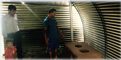
Bau & Reparatur von 40 Temporary Improved Shelter Systemen
