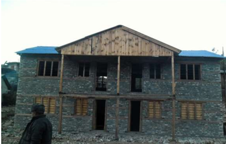
Ranukhana New School building
