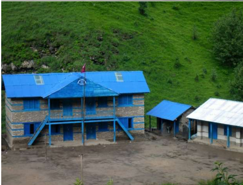
Tamti new school building (blue roof) and new toilet (blue roof)
