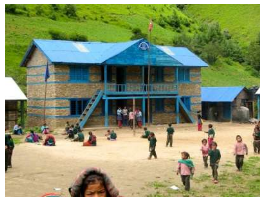
School we constructed
