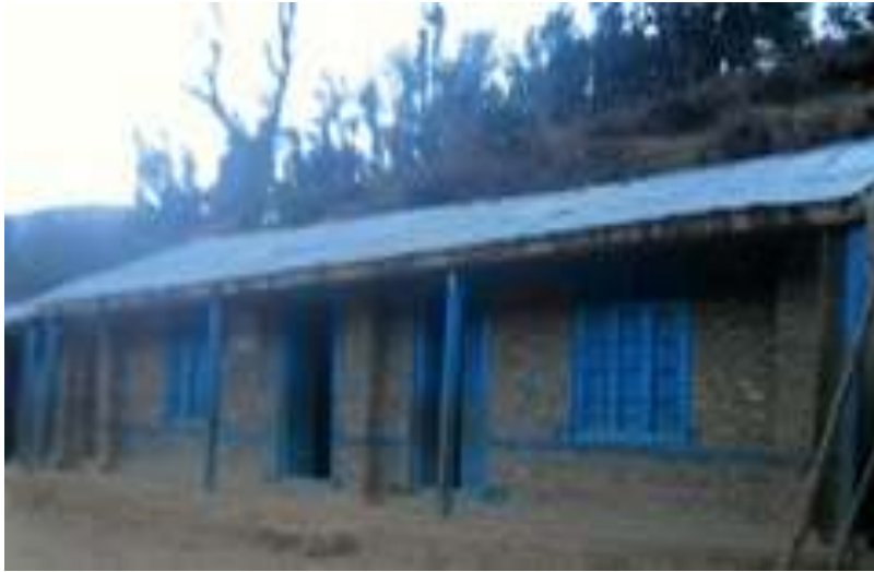
Tamti old school building
