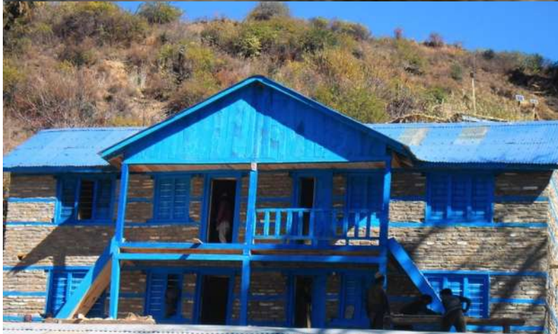
Dhipu new school building
